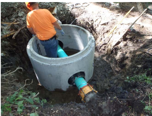
Manhole connection
