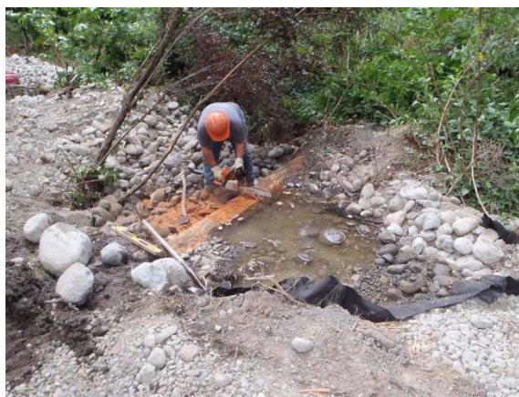
Watercourse stabilization with stream rocks and log weirs
