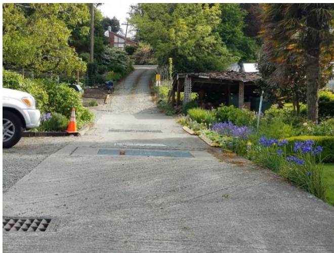
View of Freeman Avenue looking uphill east towards West Mercer Way at the top of the hill. Pavement width is approximately 15 ft. wide, ROW width is 60 ft. wide. Residential development has encroached in the entire non-paved ROW.
